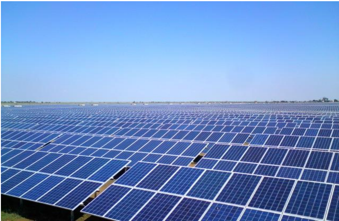
1.5 MW PV SOLAR POWER PLANT IN KARNATAK INDIA
