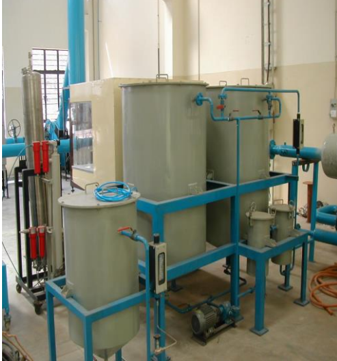
Water filtration & R.O treatment units
